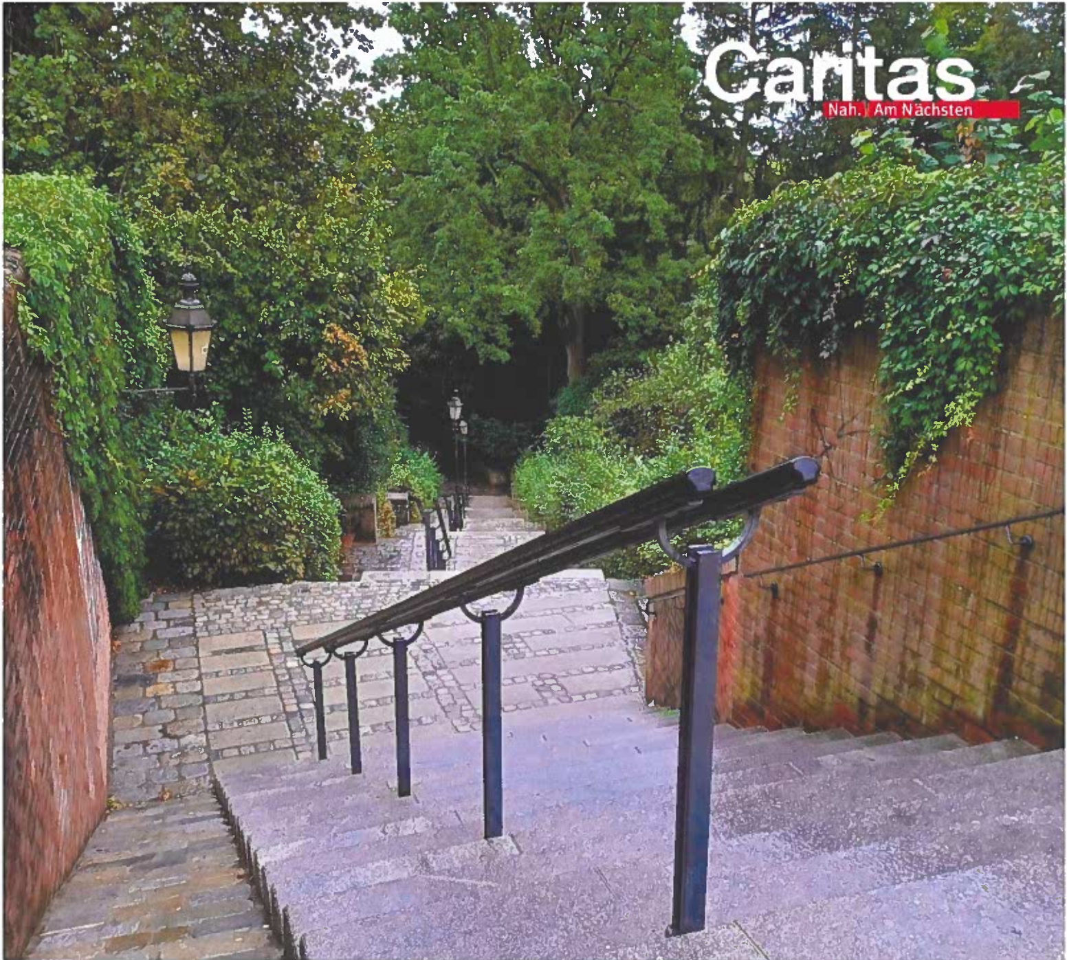
Martin Huber Treppe, Dachau
